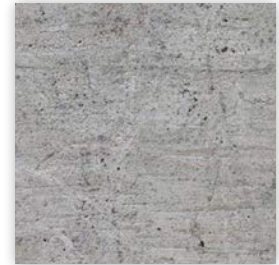
Ceiling Exposed Concrete
